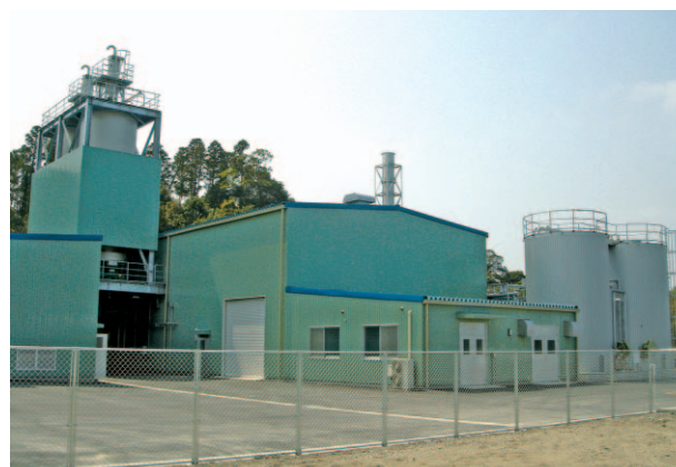
Shochu Distillation Residue Recycling Plant formerly delivered
