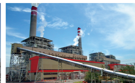
石炭火力発電所(建築土木) Marine and Land Public Work for Coal Fired Power Station
