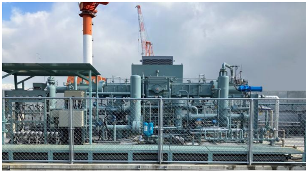
Figure 5. Pre compressor
