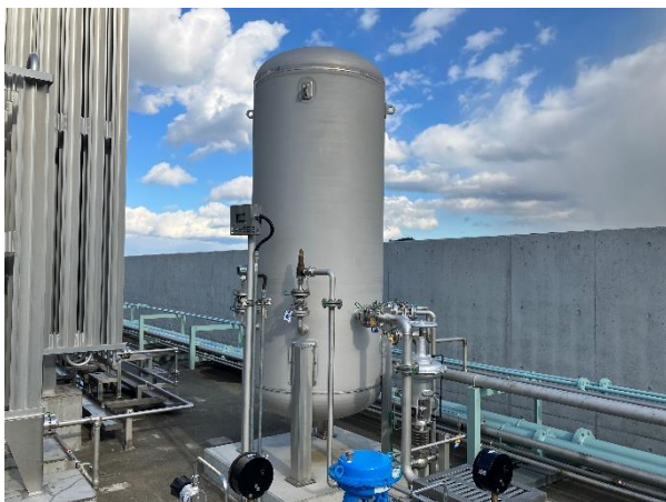
Figure 7. Buffer tank
