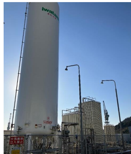
Figure 3. LH 2 Tank
