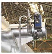
Bypass valve for EGB
