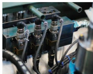
Injection control unit
