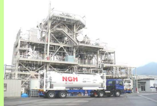
**We confirmed 5t/day of production. We will keep the evaluation of process and accumulate the necessary operational data for commercialization.**
