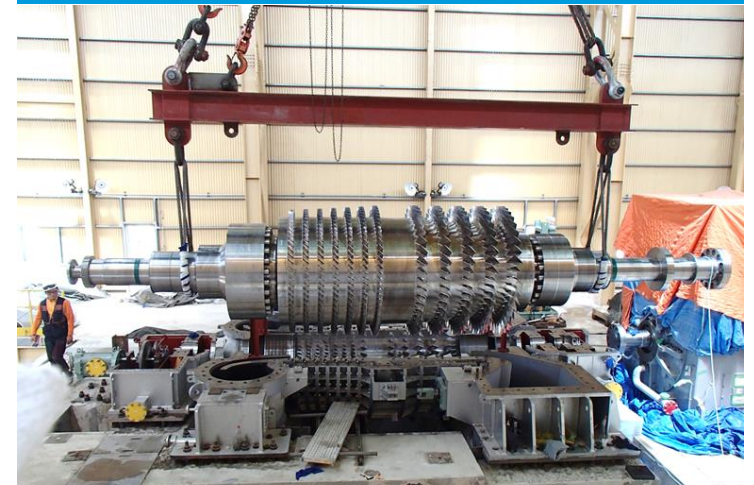
Lifting up rotor for lower casing inspection
