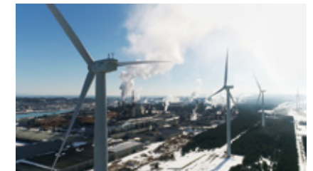
Mukaihama wind power plant
