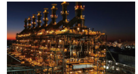
The completed cracker for the ethylene plant
