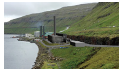
Diesel power plant for the Faroe Islands
