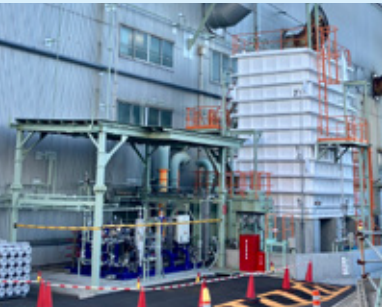
Methanol supply facilities at the Tamano factory
