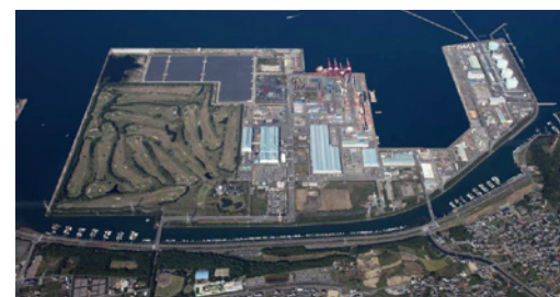
1980 – MES constructs the Oita Works in Oita City, Oita.
