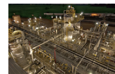
Synthetic resin manufacturing plant
