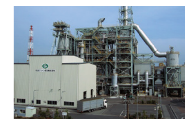
Biomass power plant
