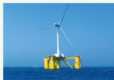
2 MW down-wind floating ocean-based power facility - Fukushima Mirai
