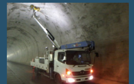
Investigation of tunnel lining concrete
